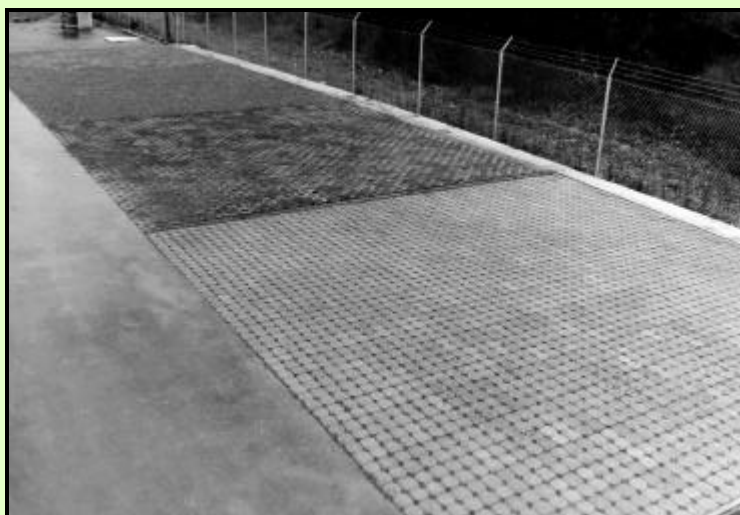
Figure 1. Different types of permeable pavement. From top left: reinforced gravel and grass pavement, reinforced grass pavement, 60% impervious concrete blocks with grass, 90% impervious blocks with gravel.
